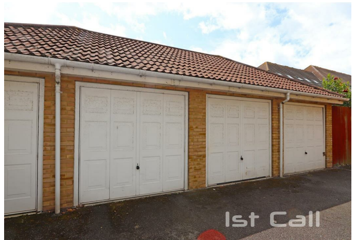
Off Street Parking & Garage
